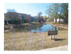
Pond #1 is approximately 4,649 SqFt in area with 307 LnFt of shoreline. The pond was dredged in 2016 at an approximate cost of \$17,000. The pond bank is lined with a concrete edging that should be effective in limiting bank degradation and silting. We have proposed an allowance of \$5,000 every seven years for pond repair and maintenance.
