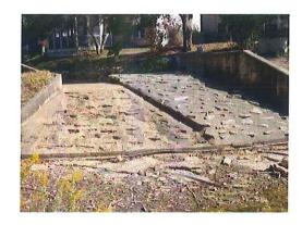
The wier that provides for flow from Pond 3 to Pond 4 has a concrete spillway and concrete sides approximately 3' high. The lifespan of the wier is indeterminate and is likely not to be replaced. We are allocating \$3,000 every 7 years for any concrete repair that would be needed.
