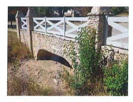
The Olde Mill Bridge is comprised of two identical structures. Each structure has four stacked stone pillars approximately 12' high with an 8' high stacked stone wall 33' in length. Additionally there is a wooden fence 3' high by 33' in length. This reserve funds the eventual replacement of the structure.
