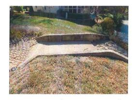
The wier that provides for flow from Pond 2 to Pond 3 has a concrete spillway and concrete sides approximately 2' high. The lifespan of the wier is indeterminate and is likely not to be replaced. We are allocating \$2,000 every 7 years for any concrete repair that would be needed.
