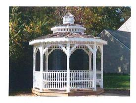
The gazebo is an octagon shaped white wood structure on a 10' diameter concrete slab. There are benches on seven of the sides with decorative wood throughout. The roof is asphalt shingled and supported by eight posts. This reserve funds the eventual replacement of the asset.
