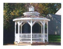
The gazebo is an octagon shaped white wood structure on a 10' diameter concrete slab. There are benches on seven of the sides with decorative wood throughout. The roof is asphalt shingled and supported by eight posts. This reserve funds the periodic refurbishment of the asset including painting, re-roofing and repairs.
