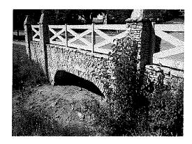
The Olde Mill Bridge is comprised of two identical structures. Each structure has four stacked stone pillars approximately 12' high with an 8' high stacked stone wall 33' in length. Additionally there is a wooden fence 3' high by 33' in length. This reserve funds the eventual replacement of the structure.
