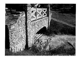
The Moss Creek Bridge is constructed of two identical structures. Each has two stacked stone columns with concrete tops 12' high connected by stacked stone walls with an average height of 8' and a length of 26'. There are wooden railings 3' high by 26' in length. To the outside of the columns are stacked stone walls with limestone caps that are approximately 10' in height and 8' long. This reserve funds the eventual replacement of the structure.
