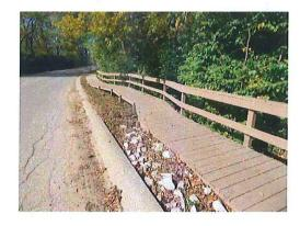
The wooden walkway is 4' wide and 210' in length with two 3' high side rails. One side rail is 210' and the second is 160'.
