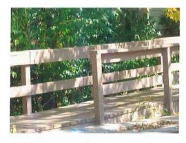
The wooden walkway is 4' wide and 76' in length with two 3' high side rails.
