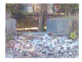
There is a concrete and rock formed dam at the outflow of Pond #7.
