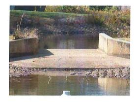
The wier that provides for flow from Pond 1 to Pond 2 has a concrete spillway and concrete sides approximately 3' high. The lifespan of the wier is indeterminate and is likely not to be replaced. We are allocating \$2,000 every 7 years for any concrete repair that would be needed.
