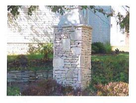
The Olde Mill Entrance is composed of a stacked stone pillar 2' x 2' x 5' high with a concrete cap. Additionally, there is a 3' high stacked stone wall that runs 150' and connects the Bent Tree Entrance Sign with this Olde Mill Entrance Sign. The cost of the stone wall is split between this reserve and the Bent Tree Entrance Sign reserve #22.
