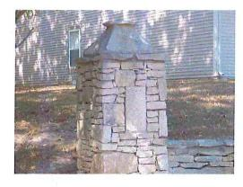
The Bent Tree Entrance is composed of a stacked stone pillar 2' x 2' x 5' high with a concrete cap. Additionally, there is a 3' high stacked stone wall that runs 150' and connects the Bent Tree Entrance Sign with the Olde Mill Entrance Sign (#24). The cost of the stone wall is split between this reserve and the Olde Mill Entrance Sign reserve #24.
