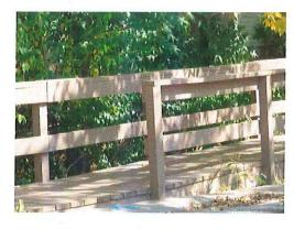
The wooden walkway is 4' wide and 67' in length with two 3' high side rails.
