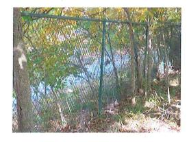
The fence then runs north to south from Graham Drive to Winslow Road for 1,236 feet There is a 6' high green chain link fence that runs south to north from Winslow Road to Graham Drive. The length of the fence is 1,236 feet. The fence appears to be in generally good condition.
